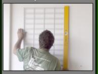
A level, a tape mesure and a drill is all you need to handle most installations.
